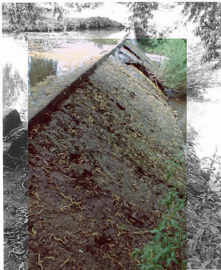
WEIR AND SPILLWAY
