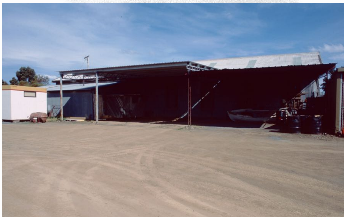
LOCOMOTIVE SHED (FORMER)
