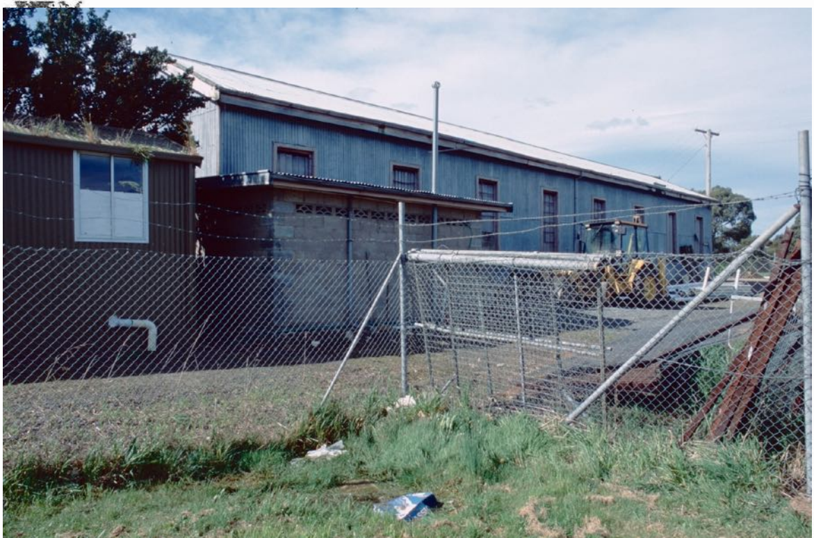
LOCOMOTIVE SHED (FORMER)
