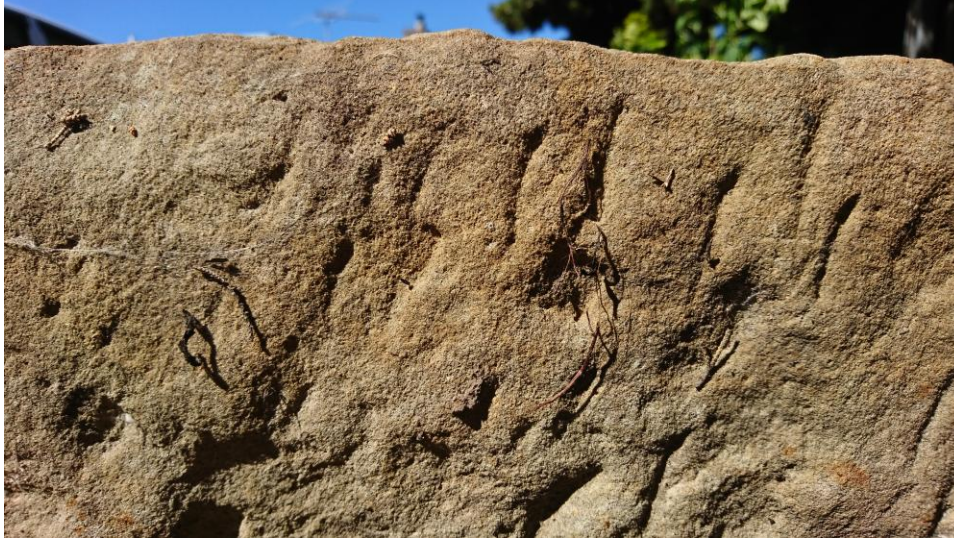
Figure 4. Chisel marks in sandstone. 9
